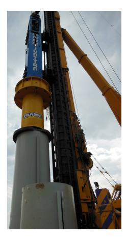
Frankipile installed over 200 steel tubes (1450mm and 1200mm diameter) which were clutched together to form the wharf's sea wall.
